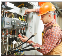
Electrician El/la Electricista
